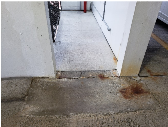
Photo 1- Rusting reinforcement
