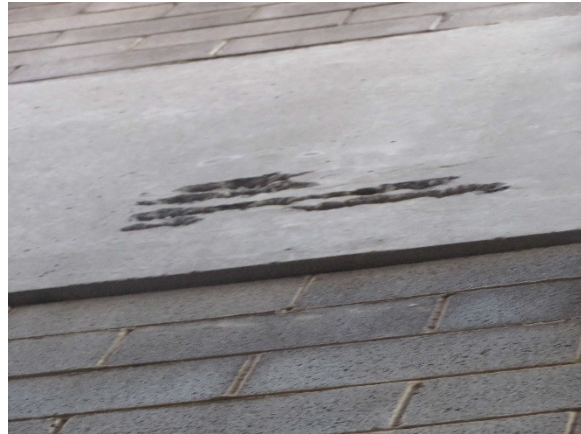
Photo 32- Spalling concrete
