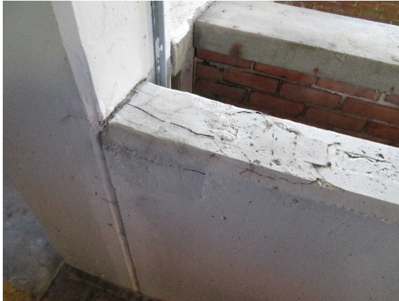
#9 – Cracked beam at top connection Level 2 Soffit grid Cx13
