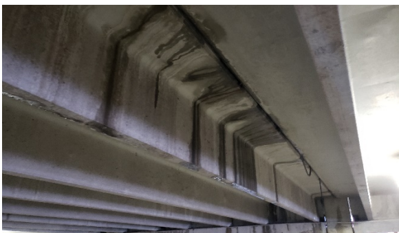
Photo 5- Leaking joint
