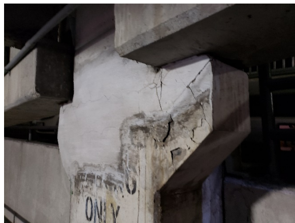
Photo 10- Cracking Column & Spalling corbel
