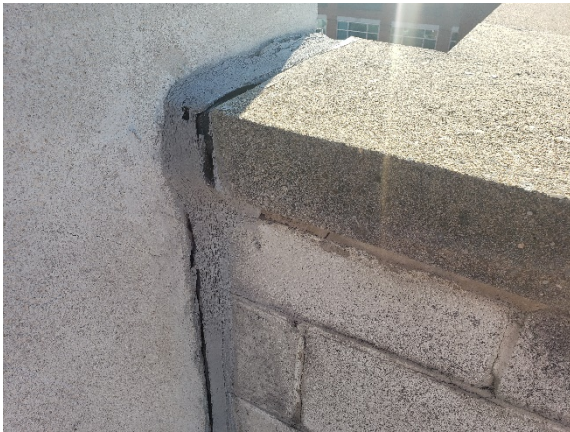
Photo 19- Failed caulk
