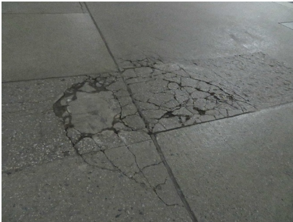
Photo 13- Spalling concrete slab
