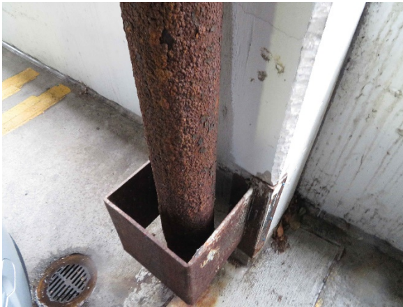
Photo 29- Corroded pipe
