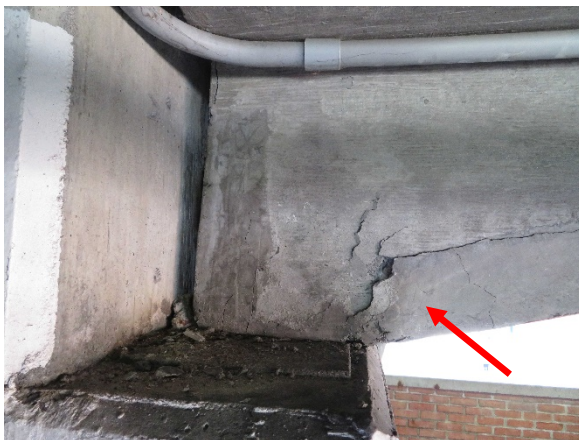
Photo 19- spalled beam at bearing
