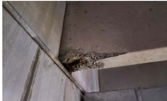
Photo 12- Spall double tee stem
