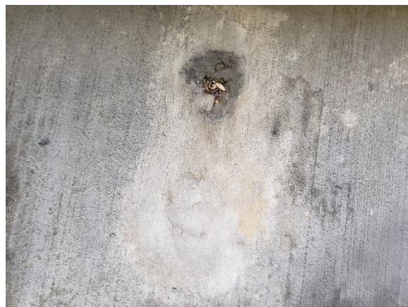
Photo 2- Spalled Concrete
