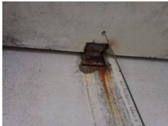
Photo 6- Spalled Concrete
