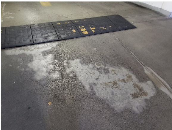
Photo 13- Worn membrane
