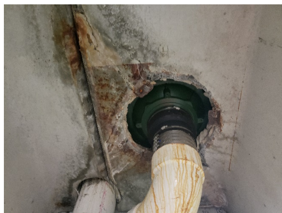
Photo 16- Spalling concrete around drain
