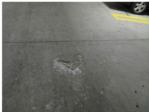
Photo 14- Spalled Concrete
