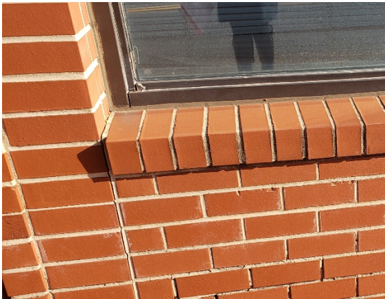
Photo 24- Failed window sealant
