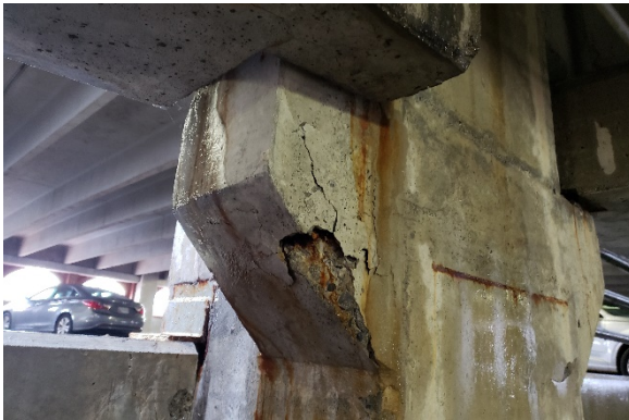
Photo 7- Rusting reinforcement & spalling corbel
