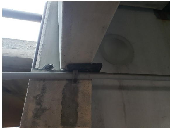
Photo 10- Failed bearing pad
