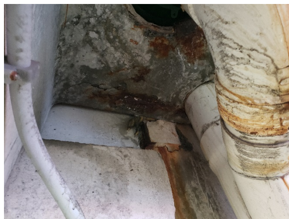
Photo 8- Spalled Concrete
