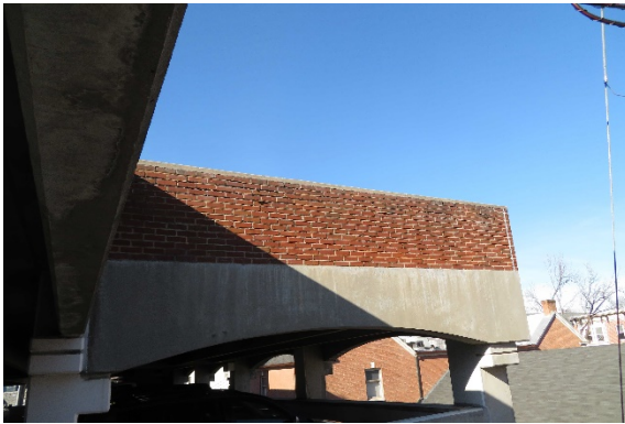
Photo 33- Loose mortar
