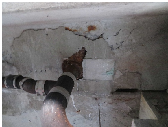
Photo 28- Spalling concrete around drain
