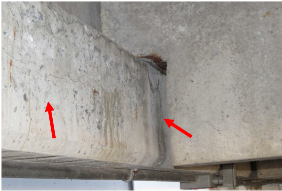
#3 – Cracked beam ledge Level 4 Soffit grid Ex9
