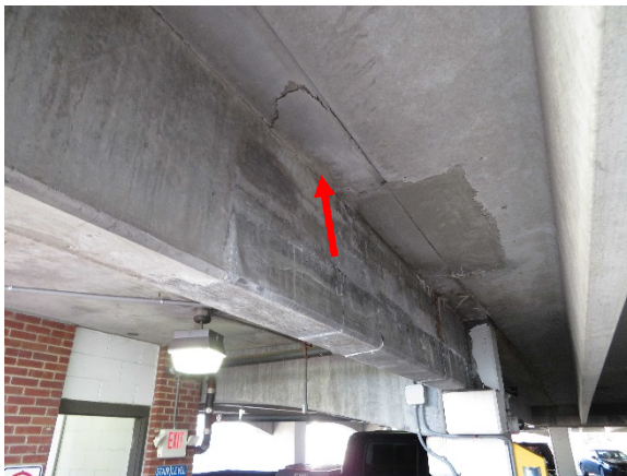
#1 – Loose concrete at beam bearing Level 4 Soffit grid Bx12
