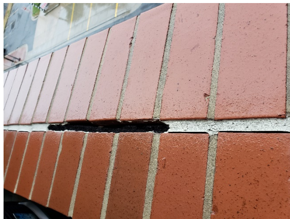
Photo 20- Failed caulk
