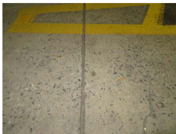
Photo 16- Scaling concrete slab
