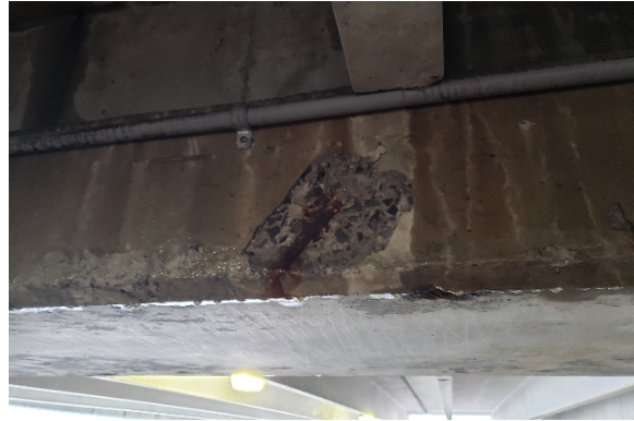
Photo 8- Spalled Concrete and exposed reinforcement
