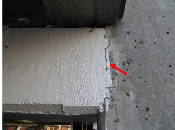
#10 – Crack at corbel Level 3 Soffit grid Ex14
