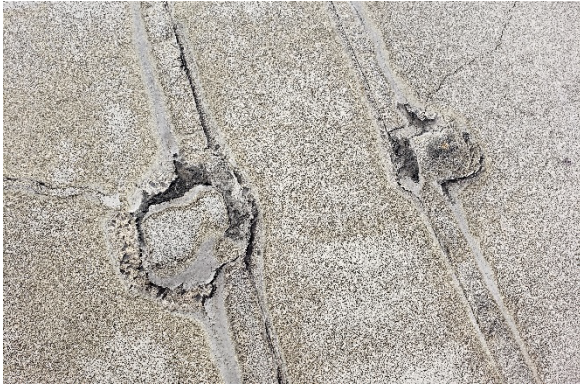
Photo 3- Spall concrete at shear connector
