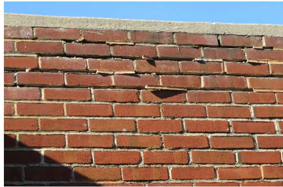
Photo 34- Loose mortar
