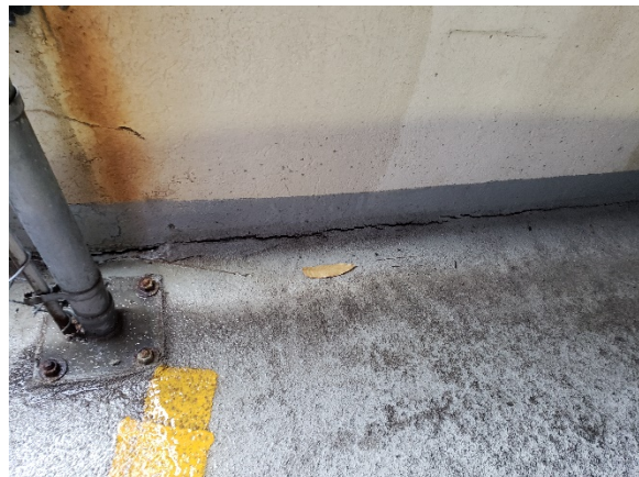
Photo 14- Cracking waterproofing membrane
