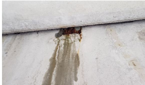
Photo 6- Spalled Concrete &amp; leaking cove joint
