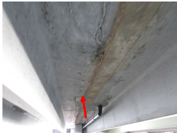
#2 – Loose concrete at DT flange Level 4 Soffit grid Dx12
