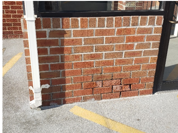
Photo 25- Deteriorated mortar joints
