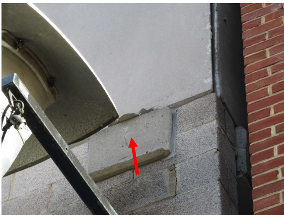
#7 – Cracked beam ledge Level 3 exterior grid Ax3
