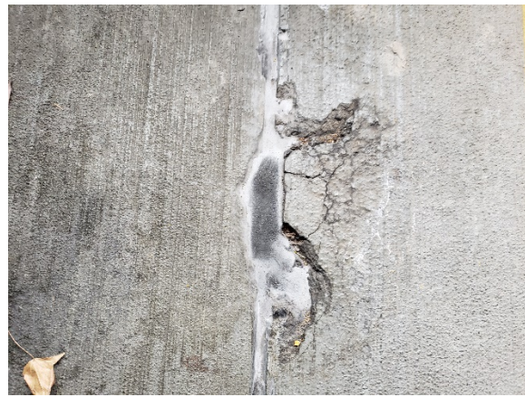
Photo 4- Spalled Concrete
