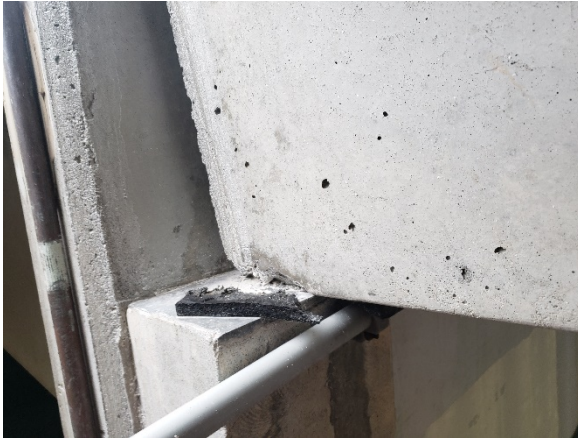
Photo 9- Failed bearing pad
