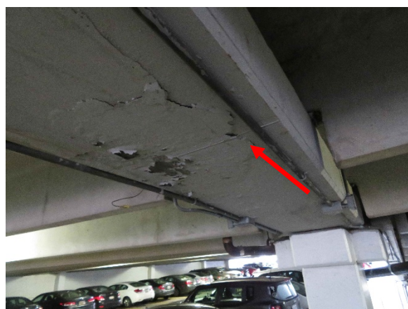
Photo 20- Spalled Concrete
