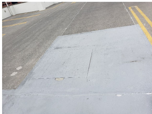
Photo 14- Failed waterproofing membrane
