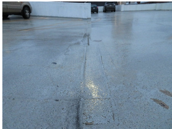
Photo 26- Exposed concrete at membrane
