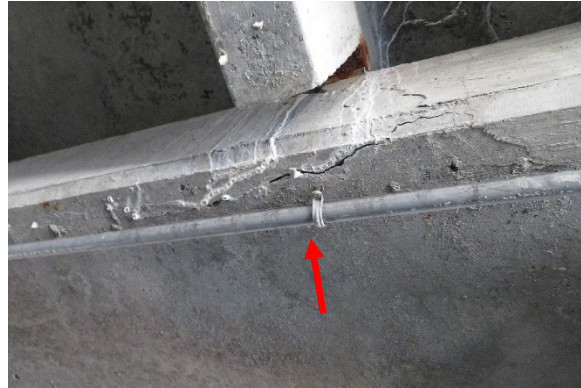
#4 – Cracked beam ledge Level 4 Soffit grid Ex12
