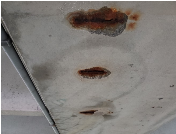
Photo 7- Rusting reinforcement
