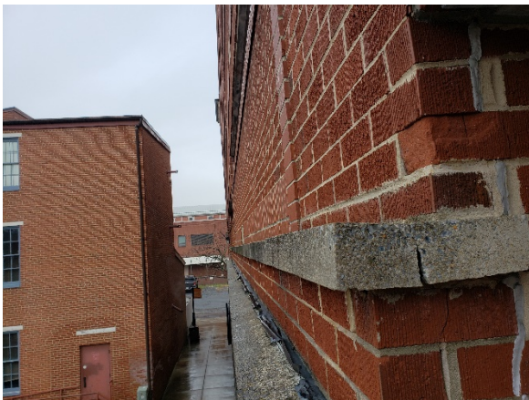
Photo 27- Cracked stone and spalled brick
