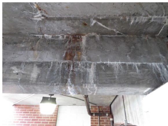
Photo 24- Cracking Column
