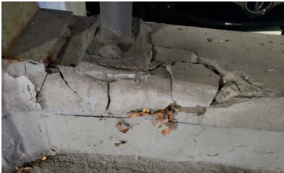
Photo 11- Spall curb
