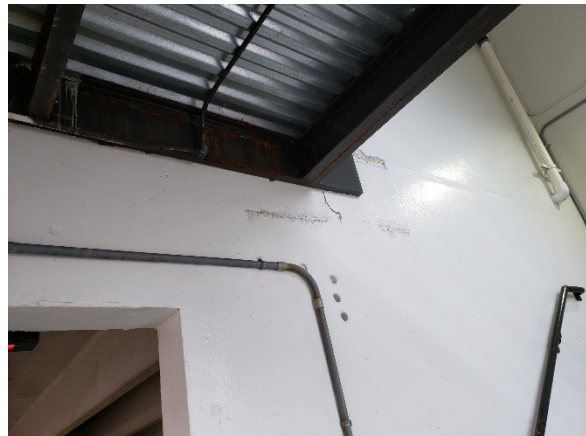
Photo 24- Slight rust on stair framing
