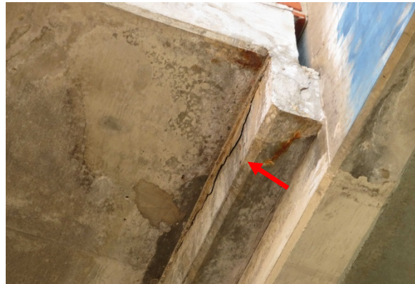
#6 – Cracked beam ledge at sliding bearing Level 4 Soffit grid Bx13
