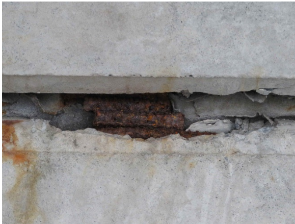
Photo 17- Rusting shear connector
