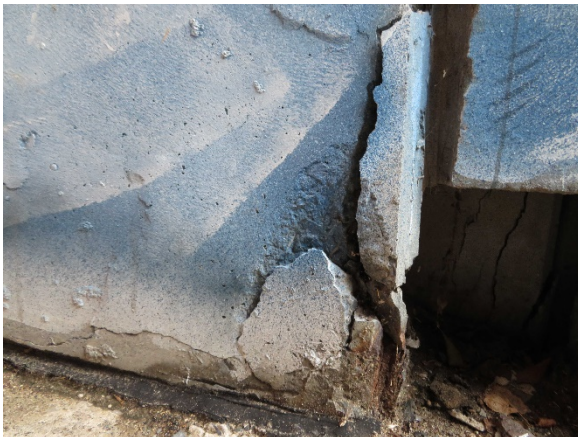
Photo 23- Spalled beam
