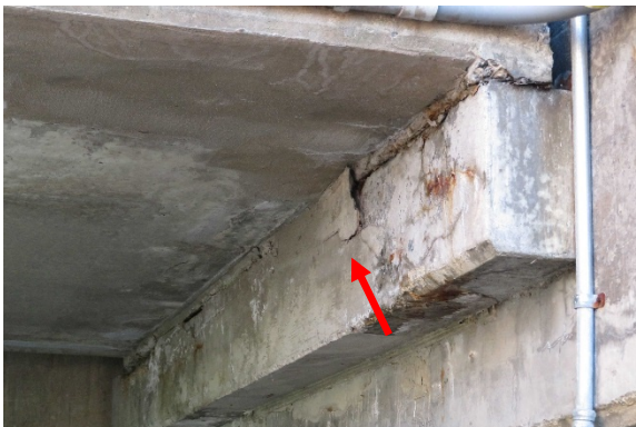
#5 – Cracked beam ledge at sliding bearing Level 3 Soffit grid Bx13
