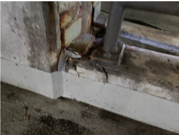
Photo 21- Rusty connection & spalled concrete
