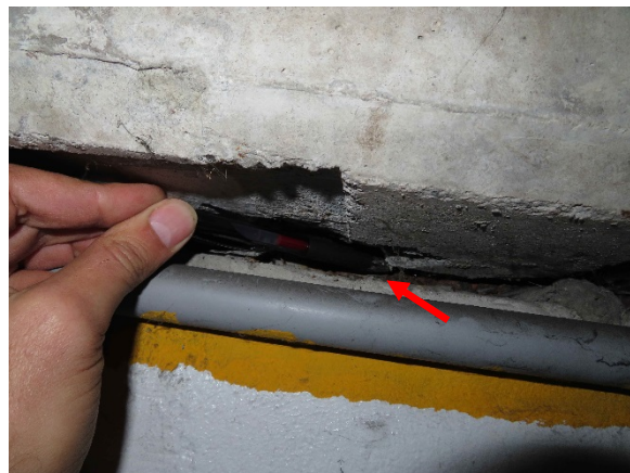
#12 – Large gap at beam bearing Level 4 Soffit grid Ex8
