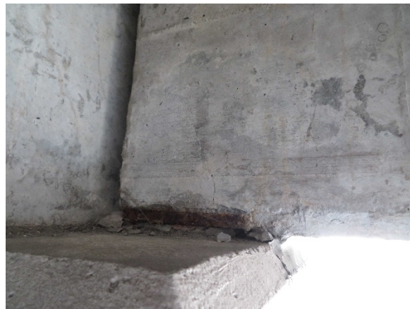
Photo 22- Failed bearing pad
