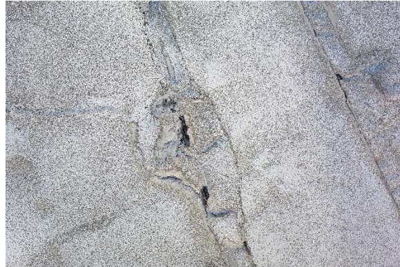
Photo 4- Spall concrete at shear connector
