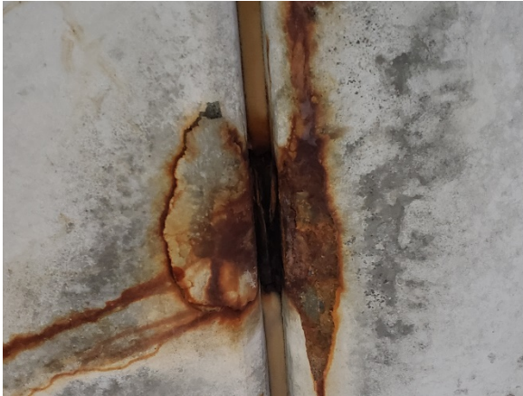
Photo 5- Rusting reinforcement
