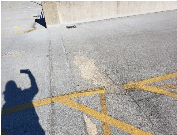
Photo 15- Failed waterproofing membrane
