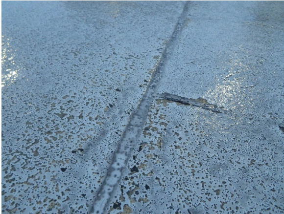
Photo 25- Exposed concrete at membrane
