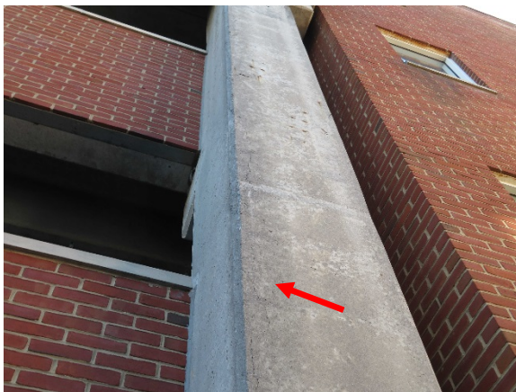
#11 – Crack at exterior column full height All Levels Exterior grid Cx14
