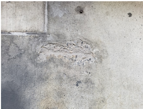
Photo 1- Spalled concrete
