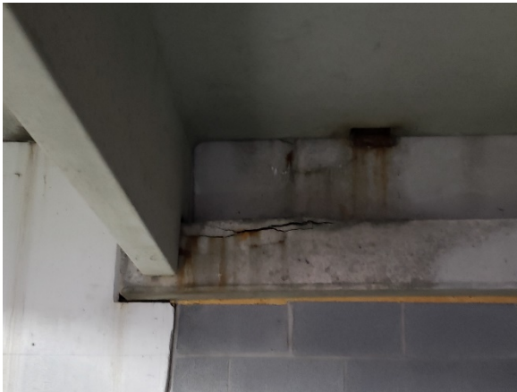
Photo 11- Spalled beam
