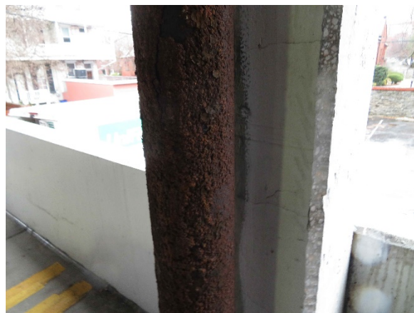
Photo 30- Corroded pipe
