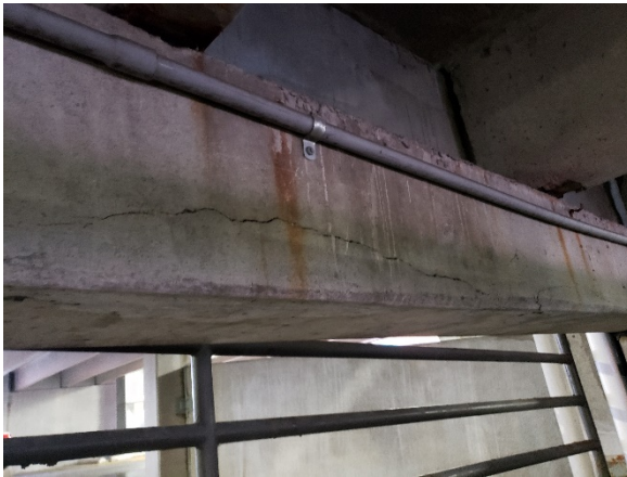
Photo 9- Spalled/cracked beam
