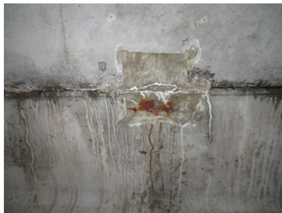
Photo 18- Spalled Concrete
