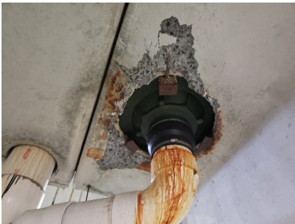
Photo 15- Spalling concrete around drain
