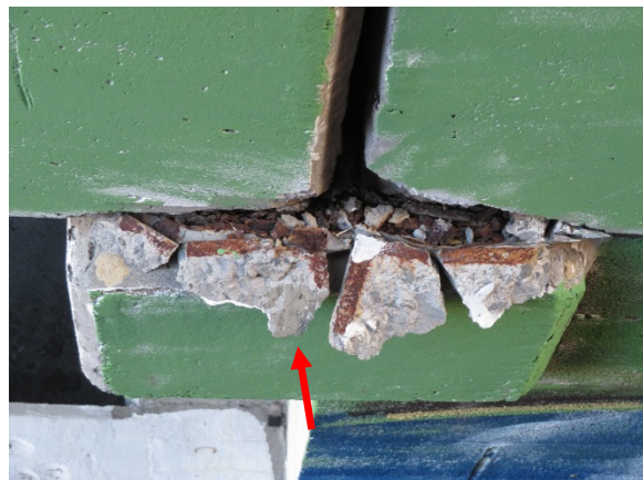
#8 – Cracked beam ledge Level 3 exterior grid Ax8
