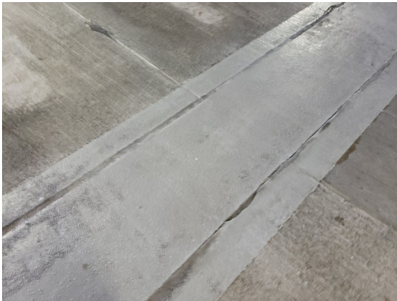
Photo 13- Cracking waterproofing membrane
